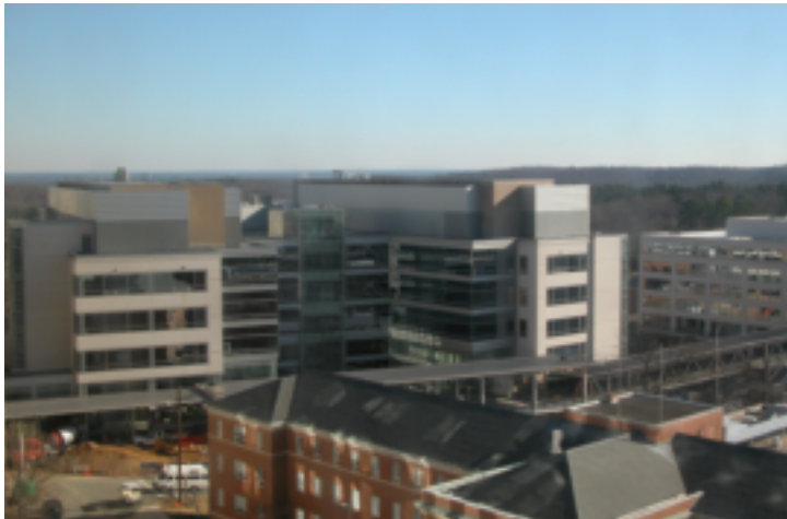
The new N. C. Cancer Hospital with Gravelly Clinical Cancer Center in the foreground and the new Physician's Office Building on the far right.
